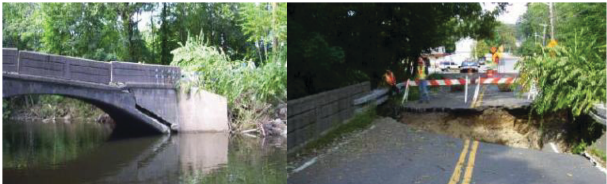
FIGURE D5 Case 7—Ramapo River Bridge damage.
